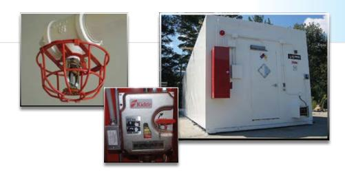
The dry chemical fire suppression system is a UL-listed, pre-engineered system rated for Class A, B and C fires with fusible link detection for automatic actuation. The automatic fusible link detectors are located on the ceiling of your building. Automatic actuation is achieved when the interior temperature reaches the desired temperature.
